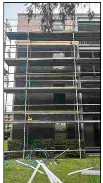
Control Joints & wire mesh building 29 stack10
