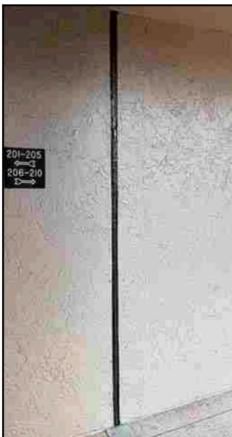
Expansion joints filled on catwalks Building 30
