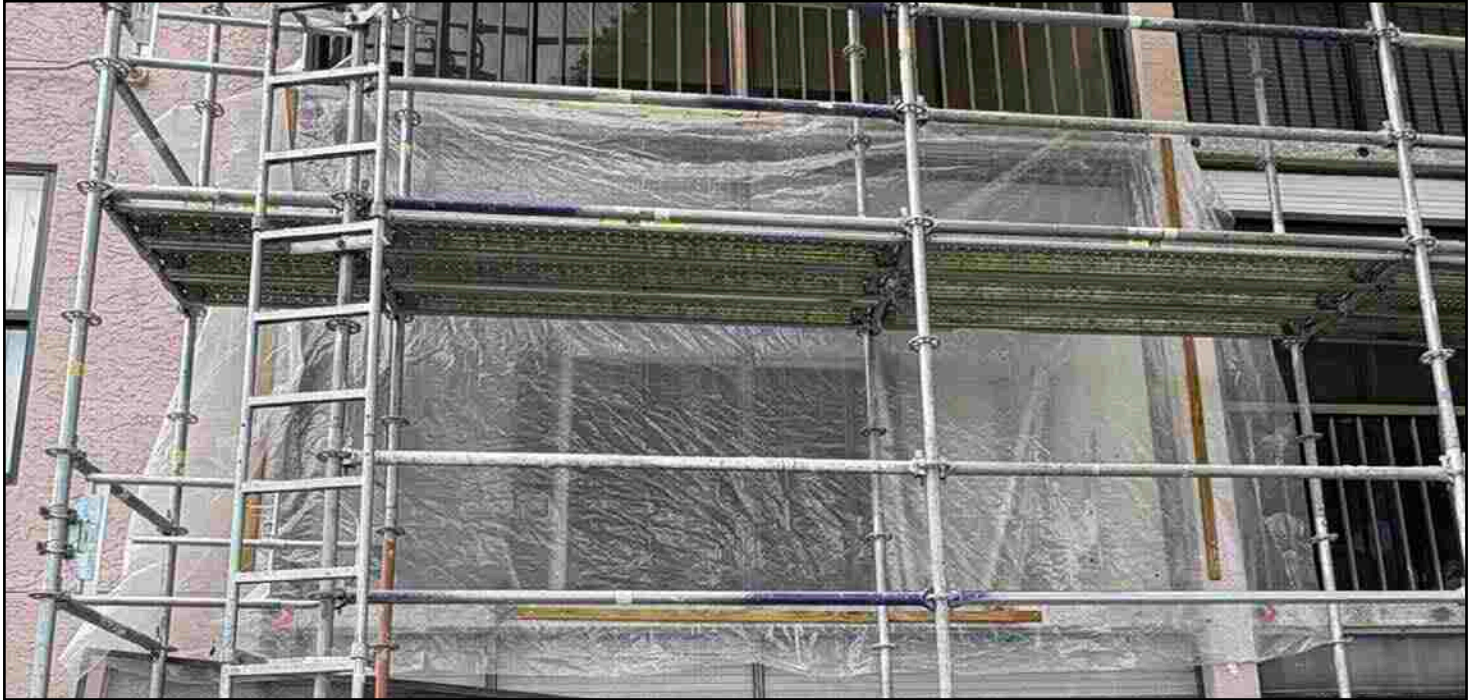
Accessories removed unit 202/bldg 30
