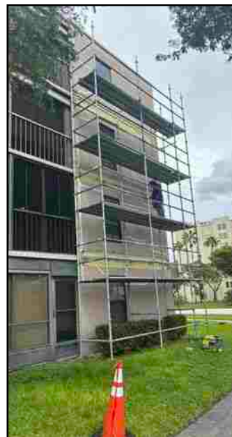
Control Joints, stack 1 building 29
