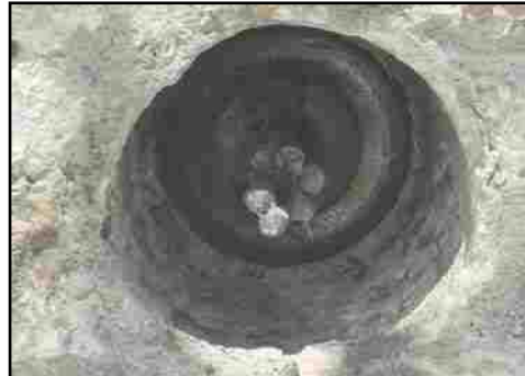
Cleaned Post tension pocket
