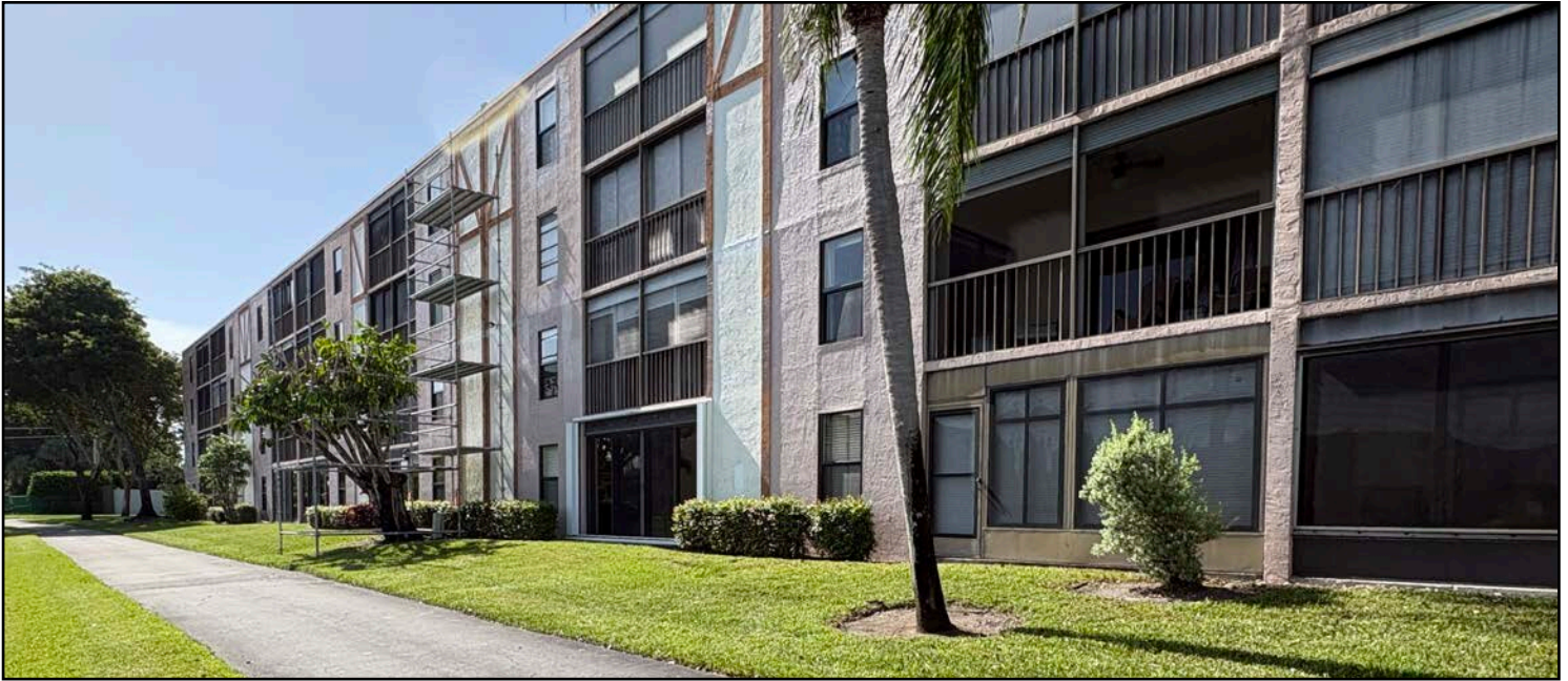
Cleanup behind BLDG 32
