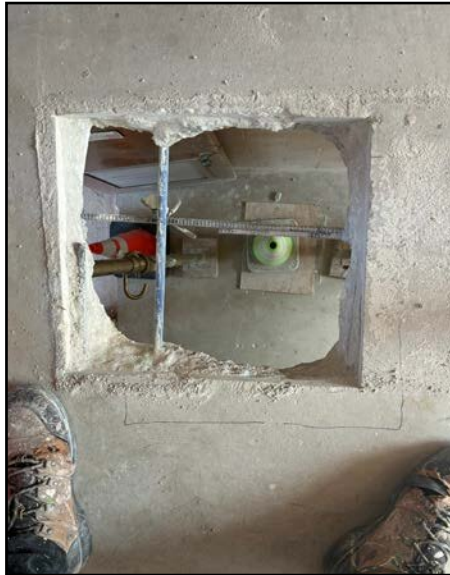
Thru Deck openings for post tension cable repairs BLDG 29
