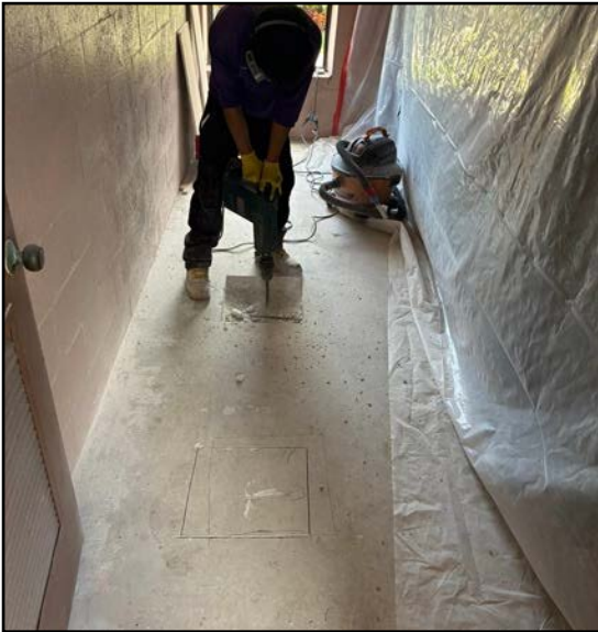
Thru Deck openings for post tension cable repairs BLDG 29
