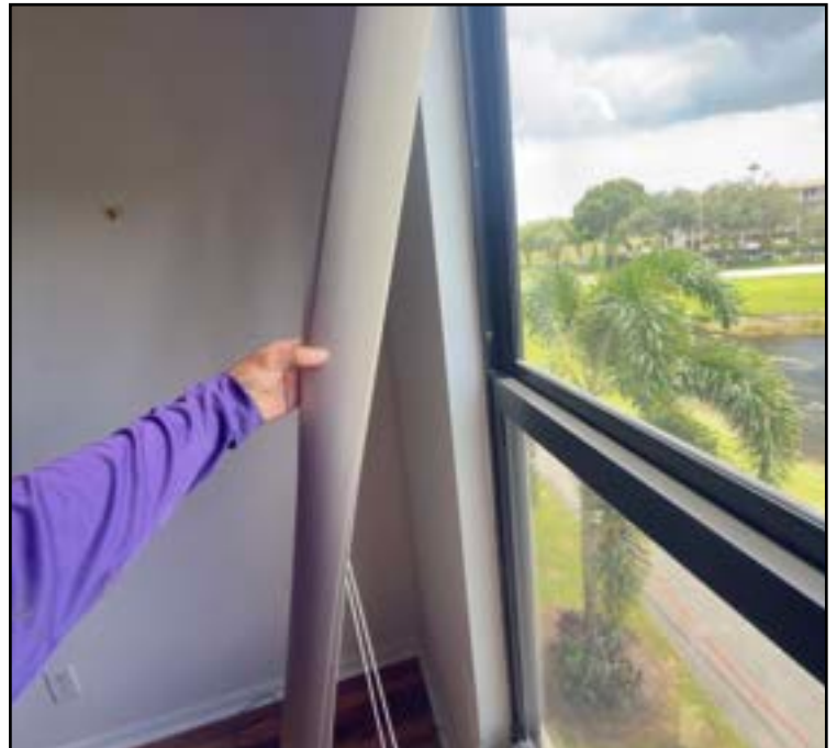
Drywall repairs, building 29
