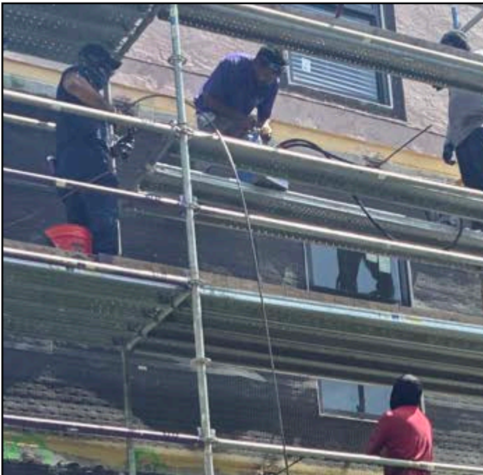
Cable stressing, building 29
