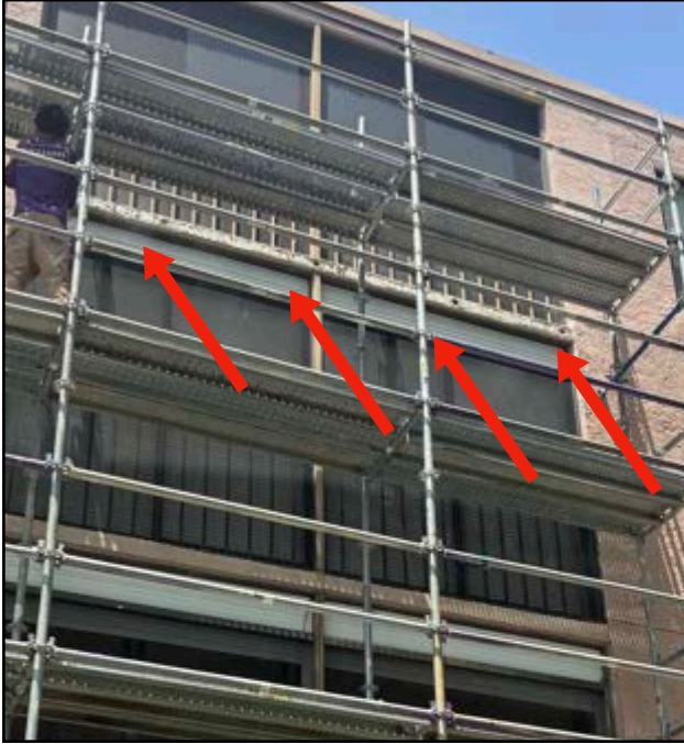
Opened PT Cable holes on building 30
