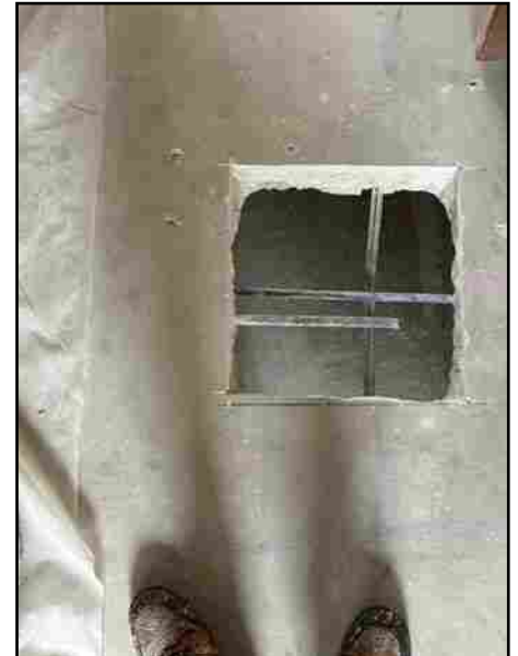
Partial depth chipping and covers BLDG 29
