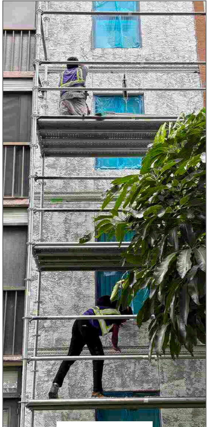
Control Joint Installation
