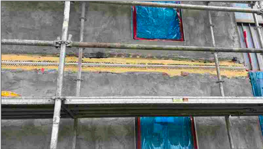
Control joints installed — waiting for inspection.
