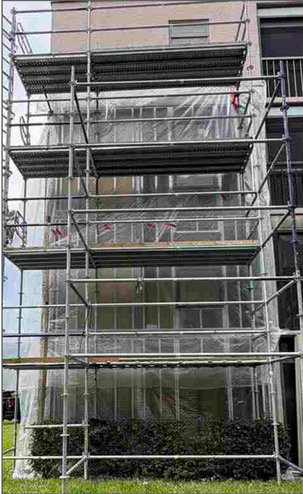
New framing on Building 29, units 101, 201, 301
