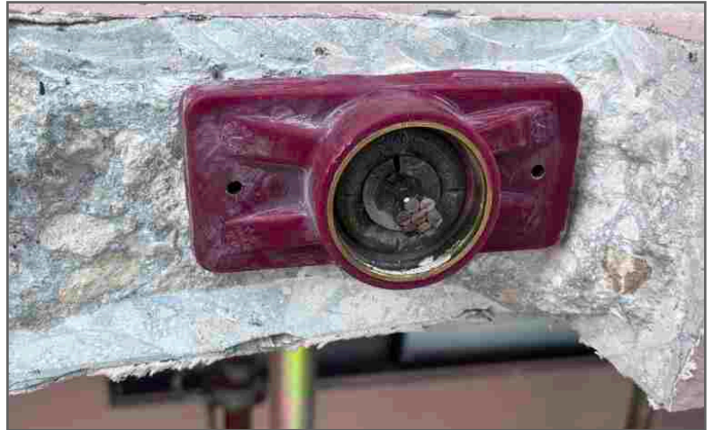
Post tension anchor repair building 30 stack 2
