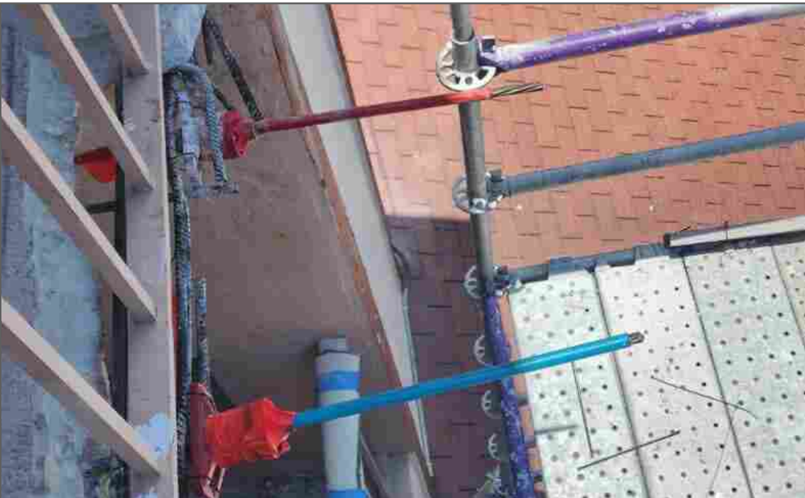
Locking off cables on building 32 by elevator
