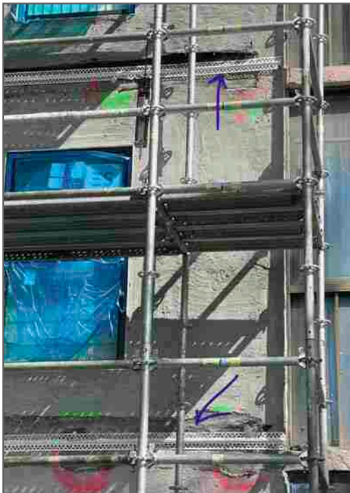
Added control joints on back of building 30
