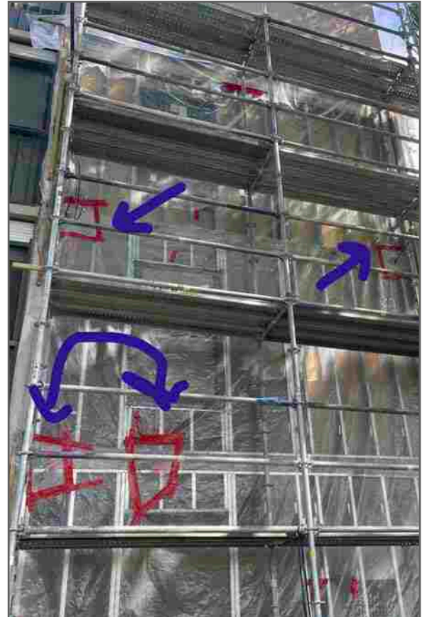
Post tension cable repairs/ replacements building 30 Stack 1
