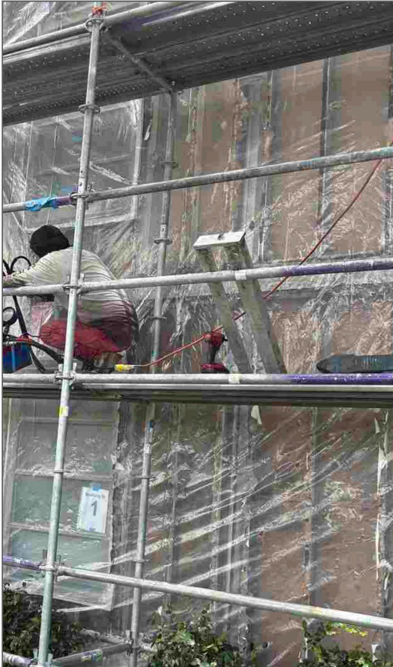
Bad wall on stack 1.
