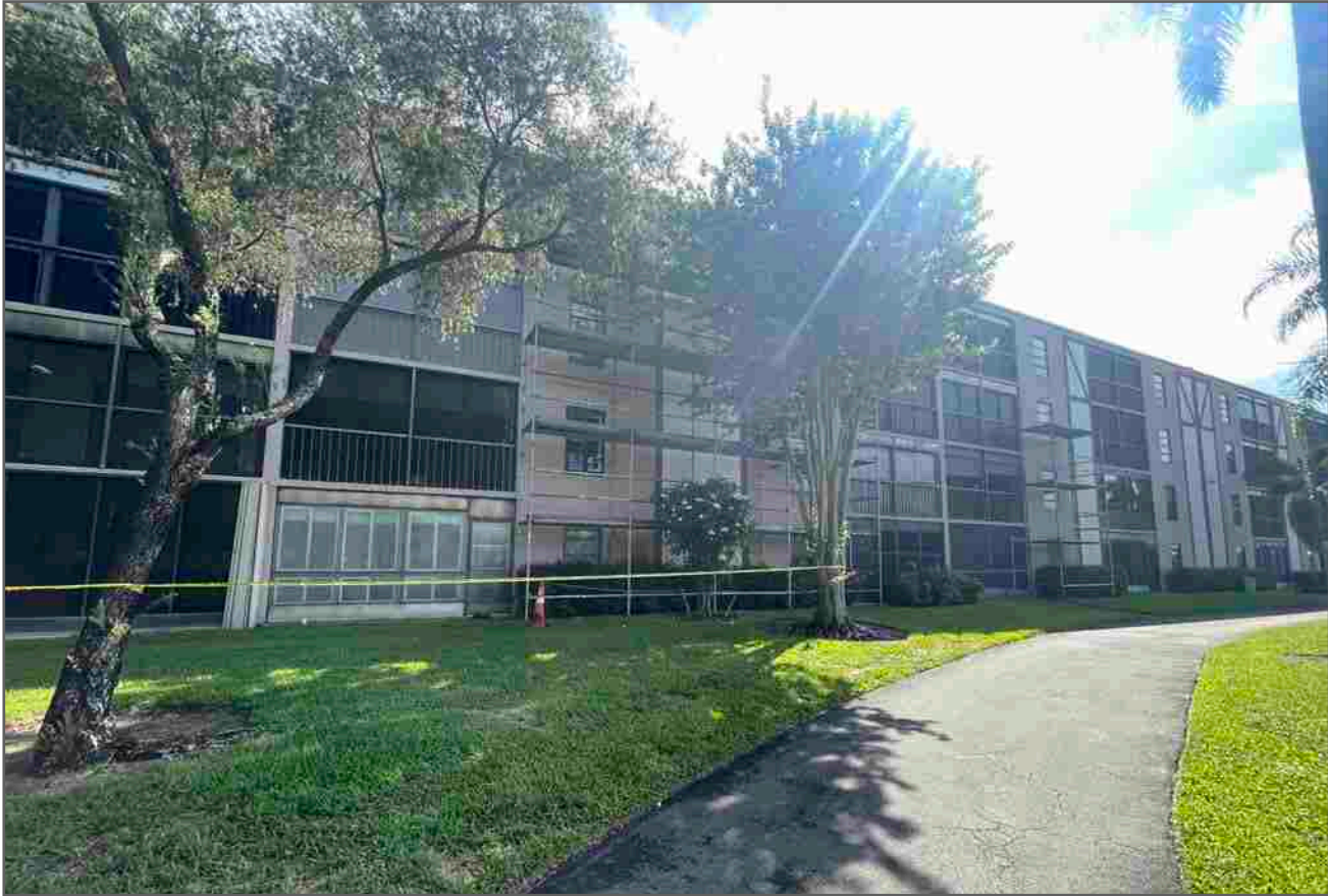
Added additional scaffolding to building 29
