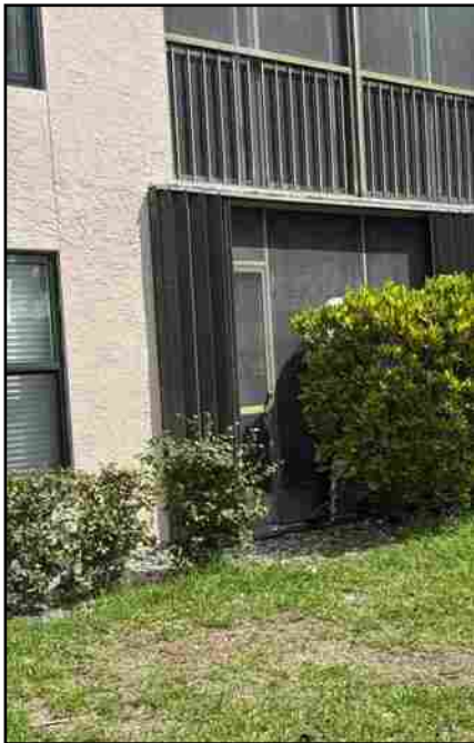
Replaced Hurricane Shutter
