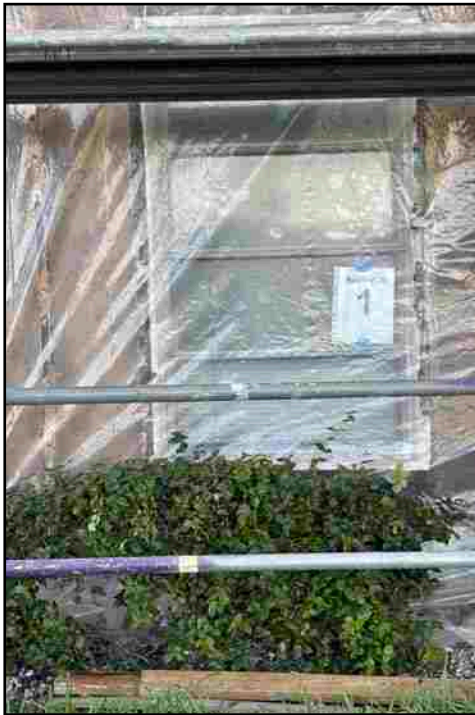
New framing 30-101. Old window reinstalled.
