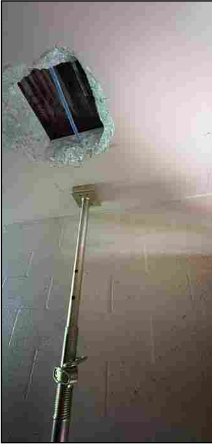
Prep for Post Tension Cable Stressing -Building 30
