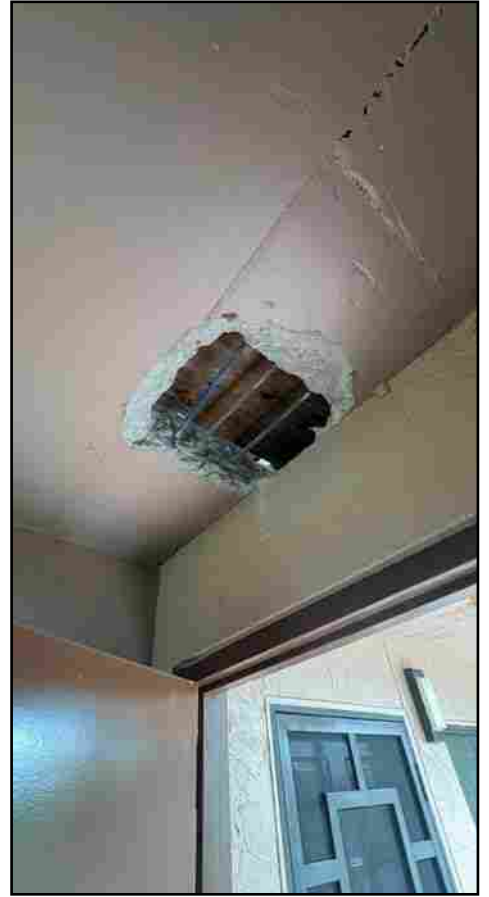
Prep for Post Tension Cable Stressing -Building 30
