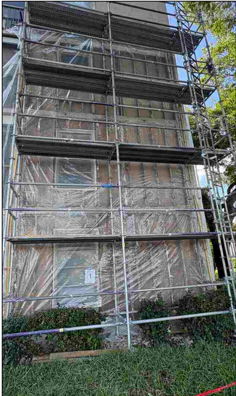
Back wall removed — one stack, building 30
