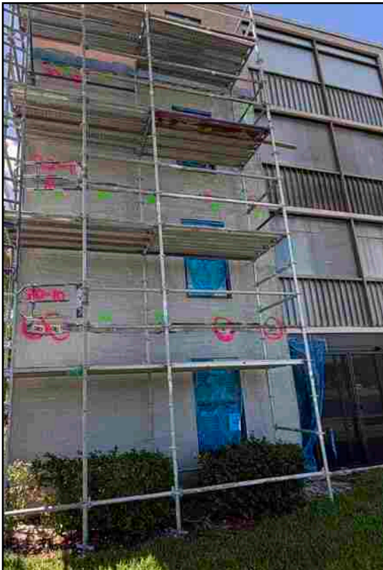
Cleaned cut and painted 25 post tension cable pockets
