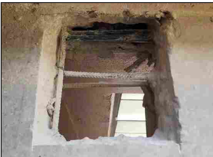
Prep for Post Tension Cable stressing Railing post pocket concrete pours
