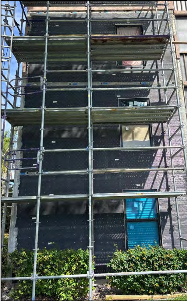
Wire mesh installed.
