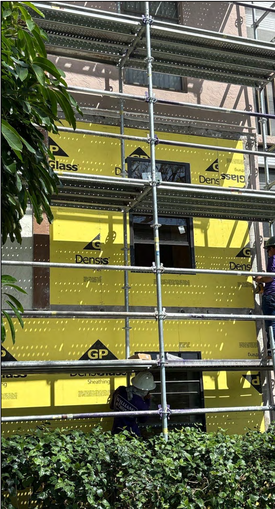
Dens Glass installation
