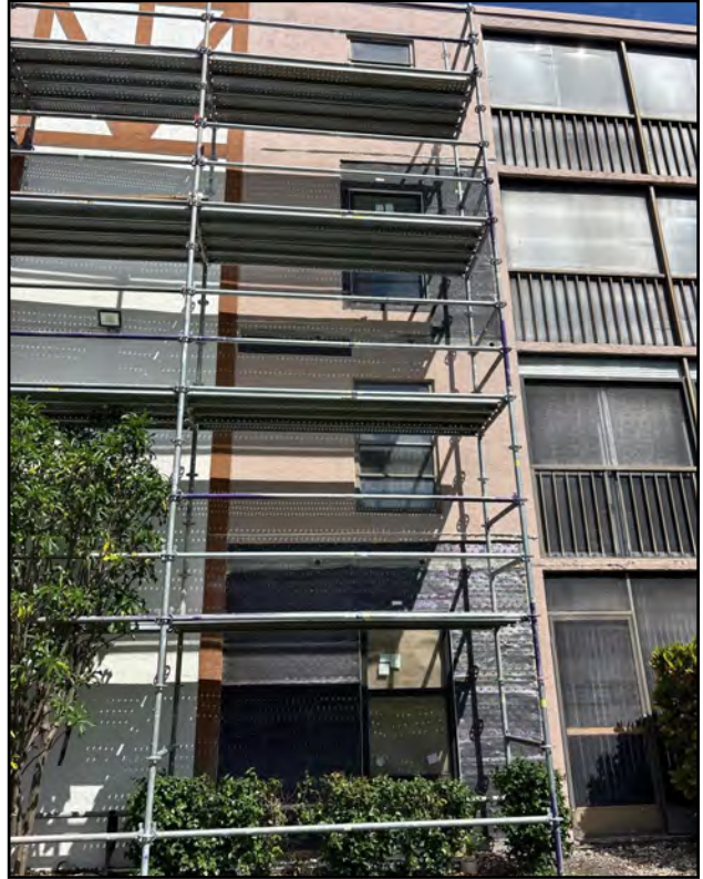
Wire mesh installed.
