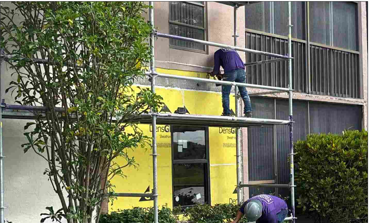
Dens Glass install
