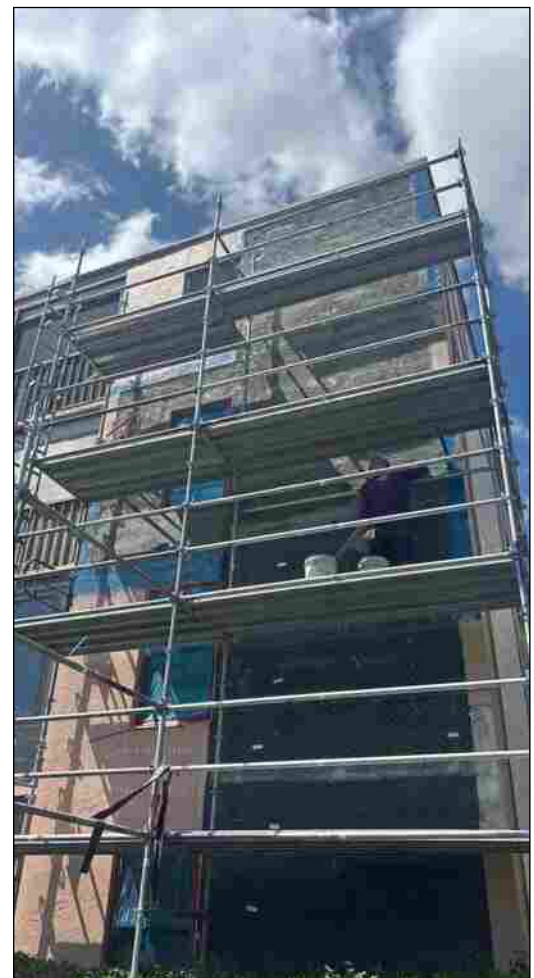
Installation of wire mech on dens glass wall on building 31
