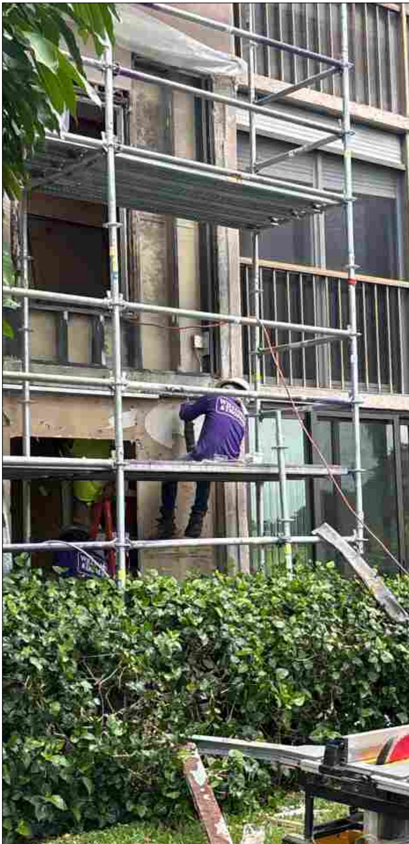
Installation of plywood weather walls and framing work on building 30
