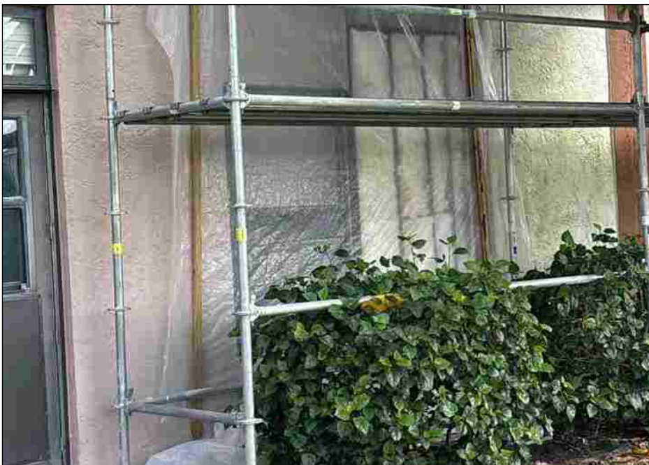
Window install, insulation and framing
