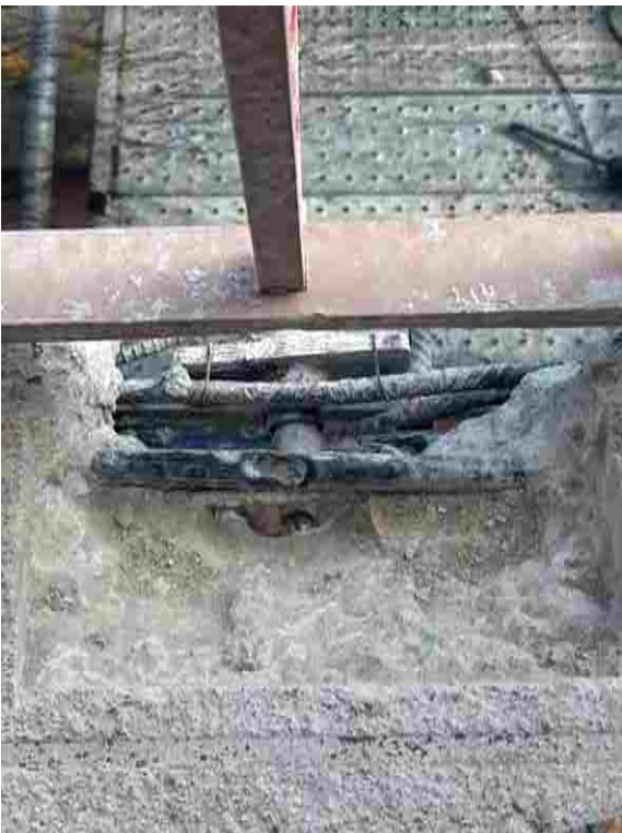
Post tension cable repair prep building 32
