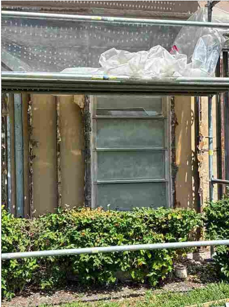
Extensive framing damage in building 30
