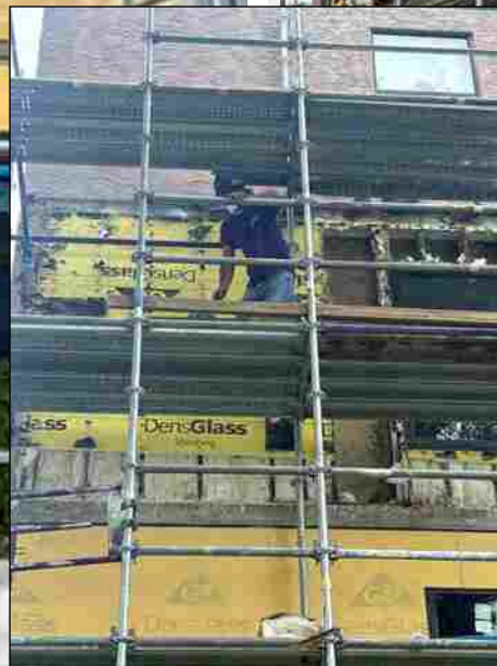
Dens Glass Installation Building 30 1 stack
