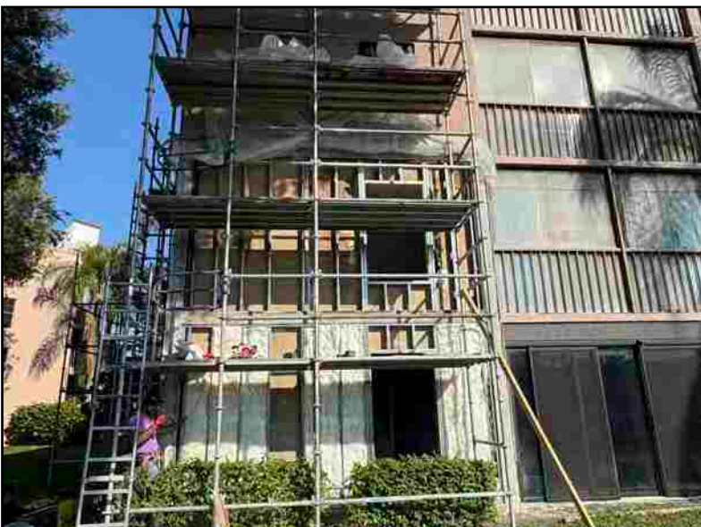
Exterior wall repairs, buildings 31 and 30
