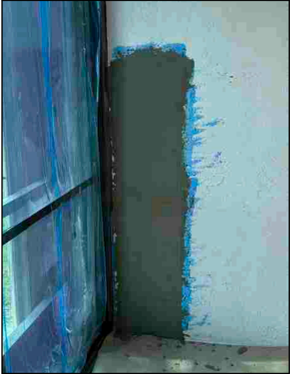
Interior repairs, building 30
