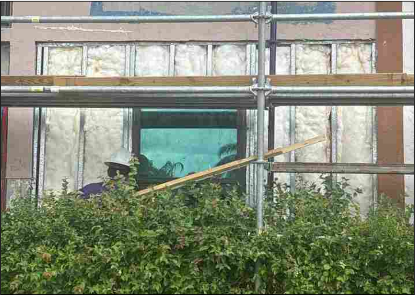
Exterior wall repairs, buildings 31 and 30
