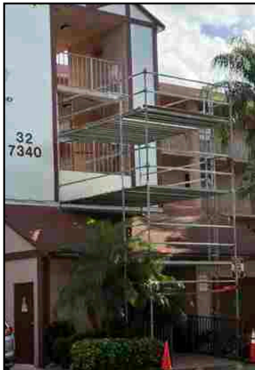
New scaffolding building 32
