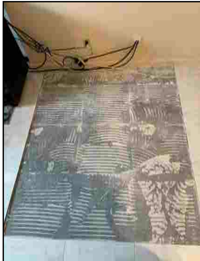
Tile removal bedroom 31/306
