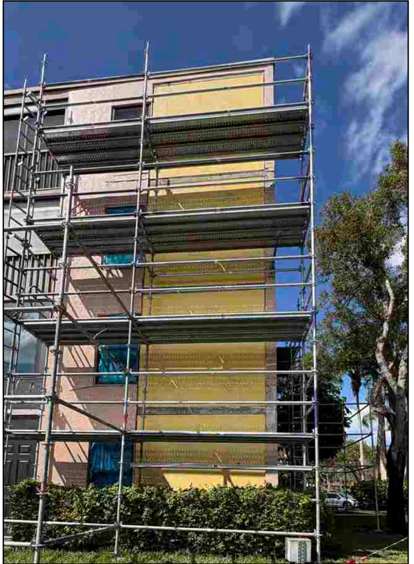
EFIS walls on entire one stack
