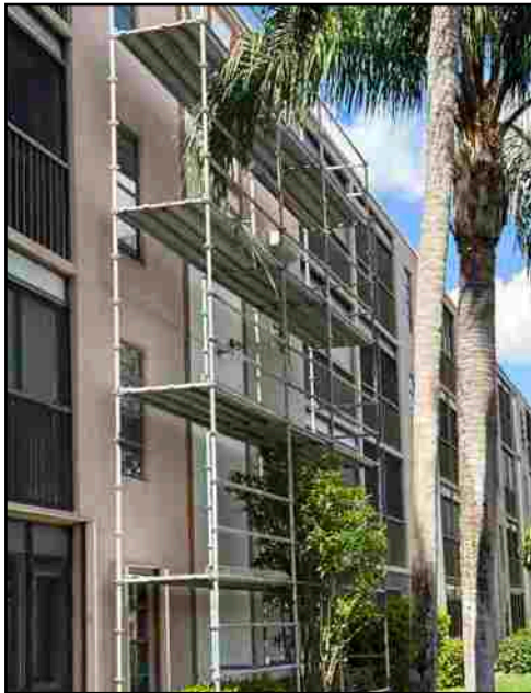
New scaffolding building 30
