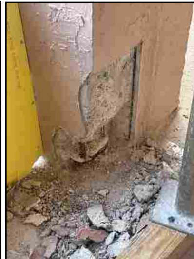
Column excavation bldg. 30
