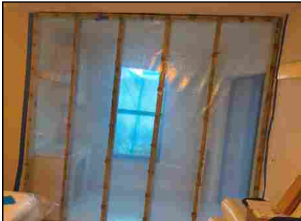
Dust walls installed — buildings 31 and 30
