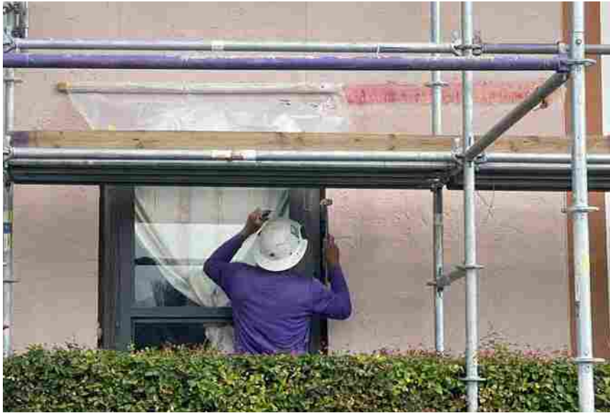
Window Protection and Dens Glass installation
