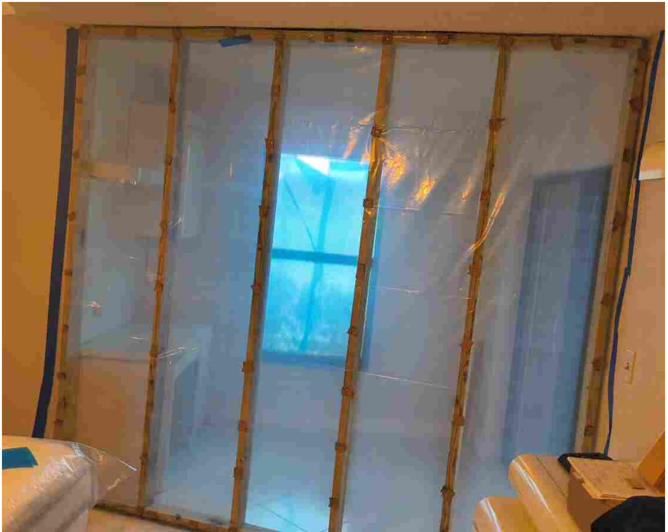
Interior dust wall
