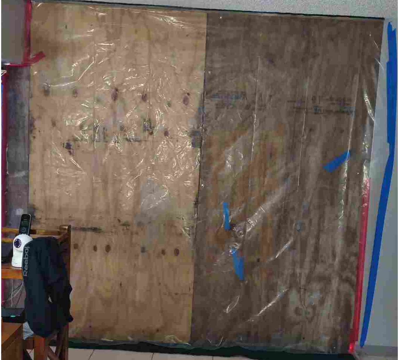
Plywood Weather Wall
