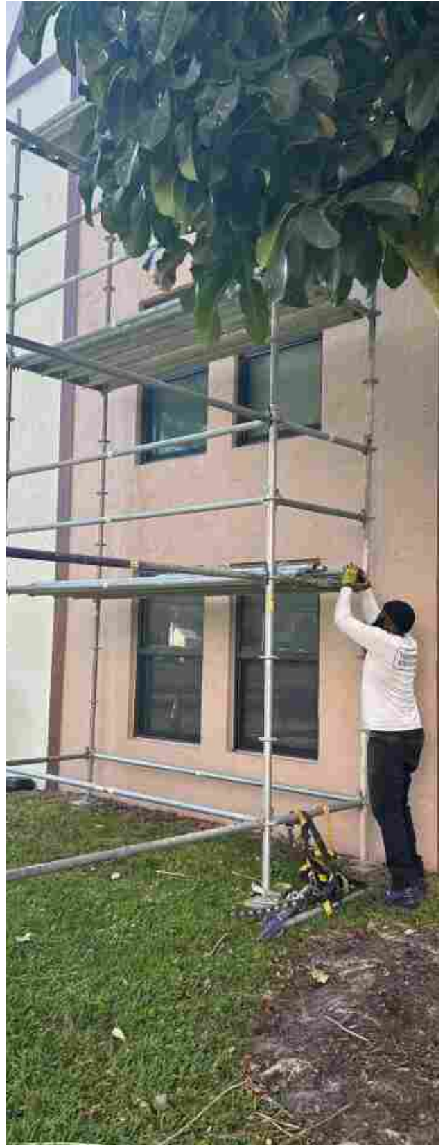
Scaffolding on building 31
