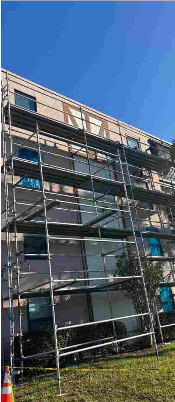
Wire Mesh installed around windows
