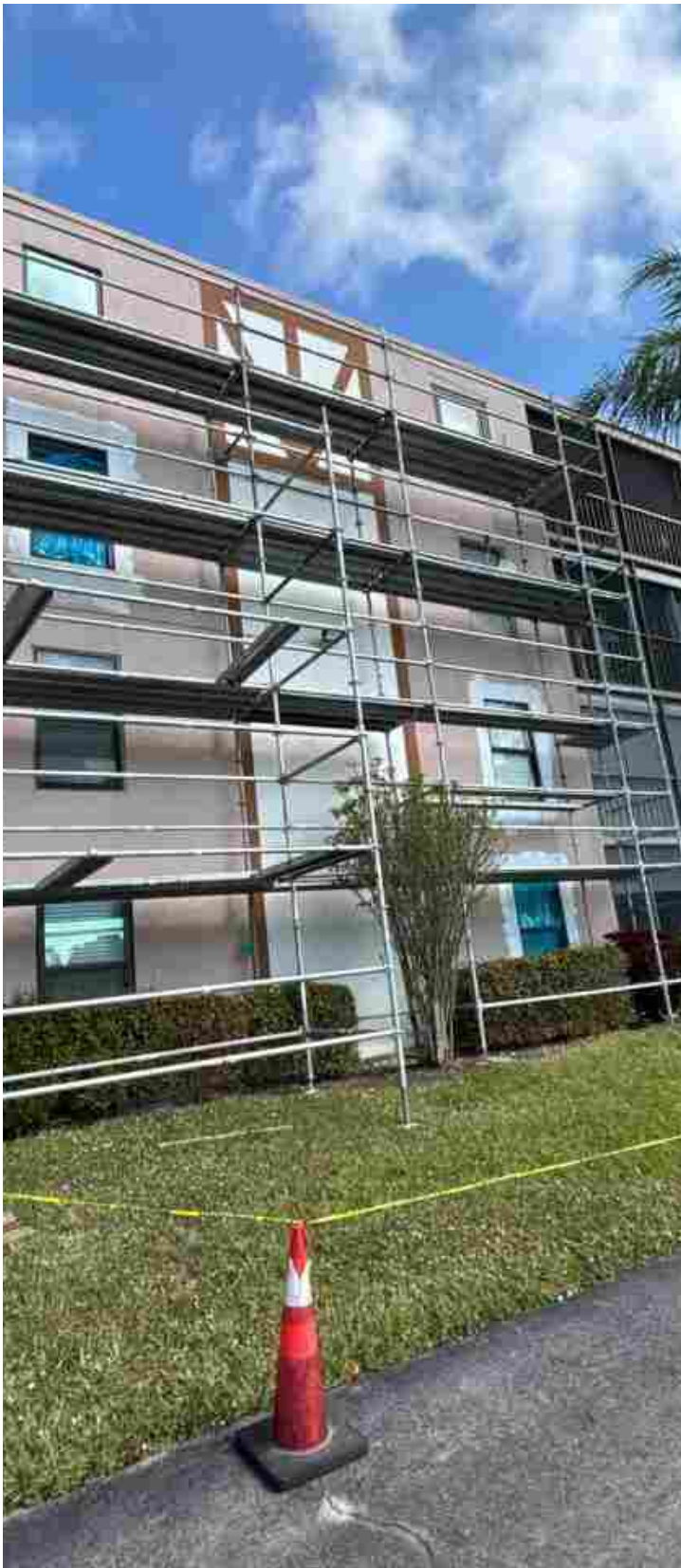
Applied primer around windows
