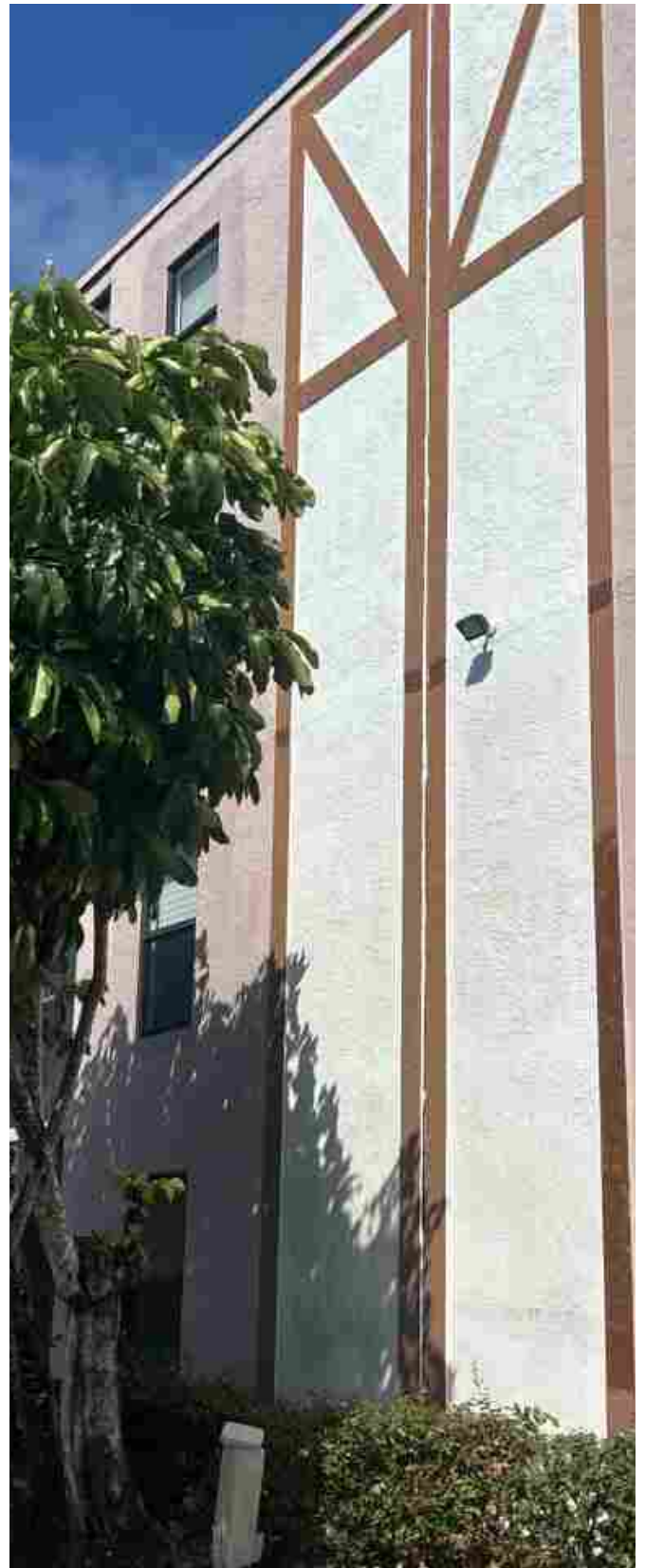
Completed EmSeal install in expansion joint on BLDG 32 South, and North elevations (third floor)
