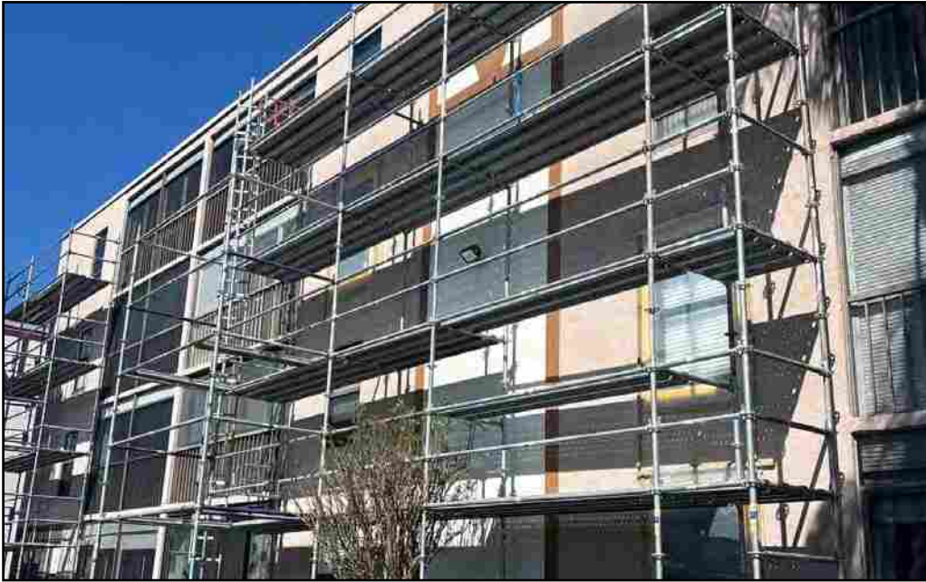
Window and Dens Glass installs south elevation BLDG 31
