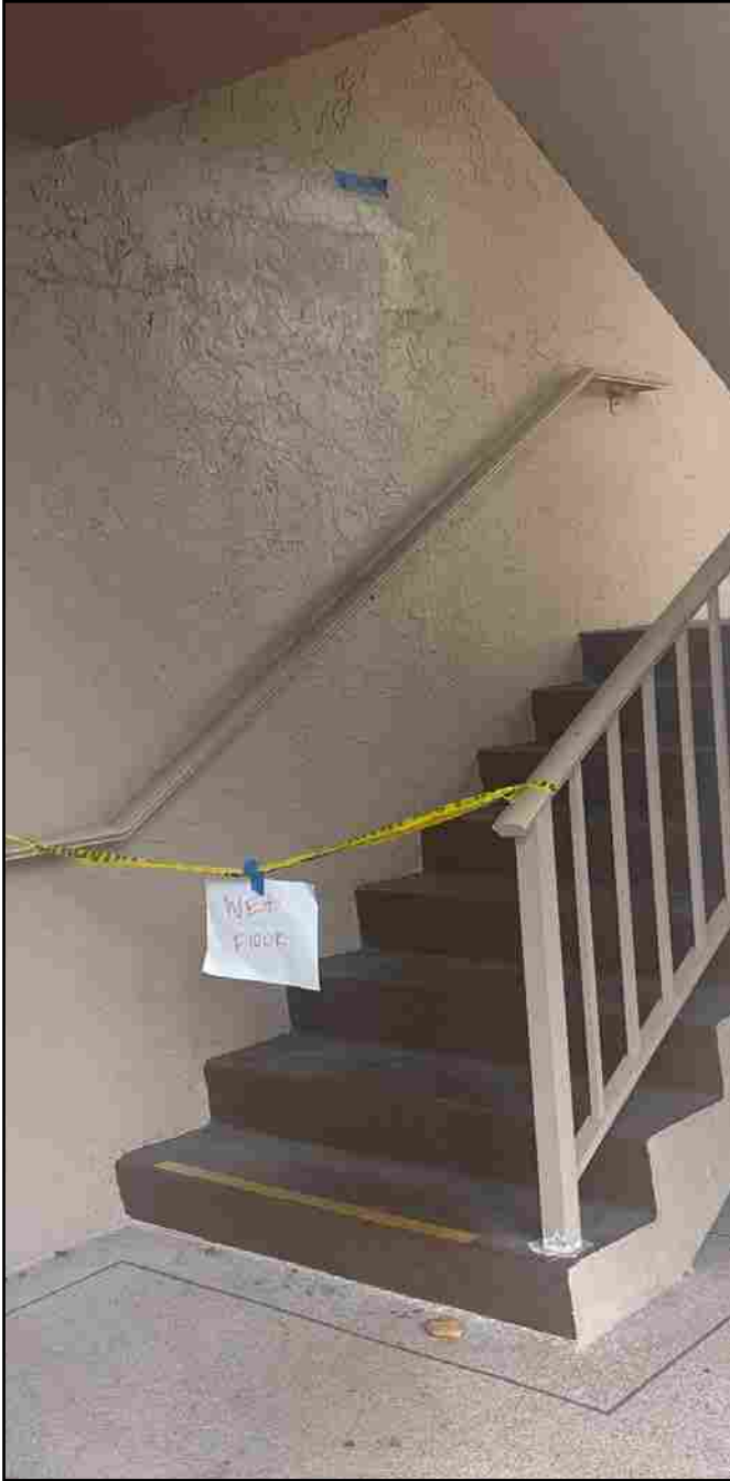
Painting in stairwell Building 32
