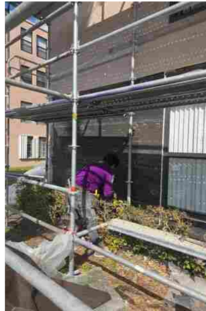
Wire mesh, Stucco and paint on EFIS wall South Elevation BLDG 31
