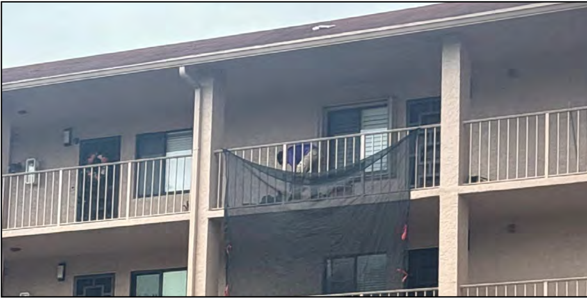
Chipping post pockets. Fourth Floor Bldg. 30
