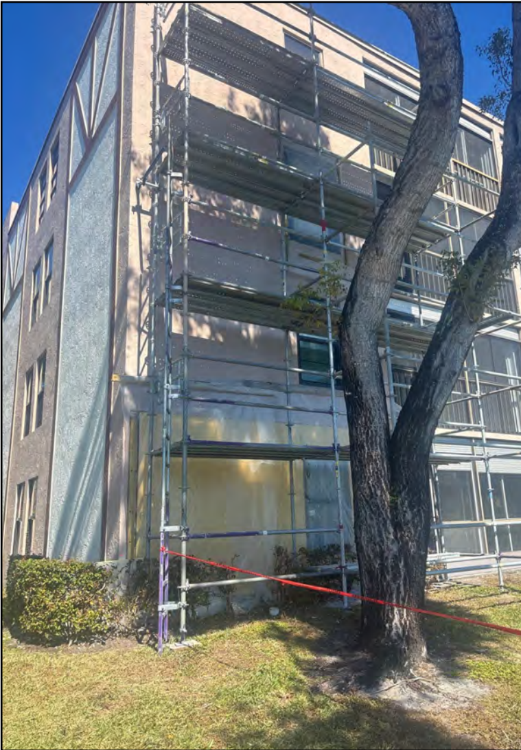
Dens Glass installation
