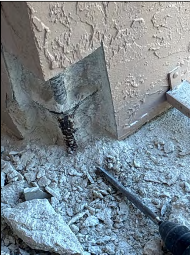
Column Excavations Building 30
