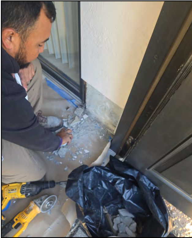
Interior Stucco work
