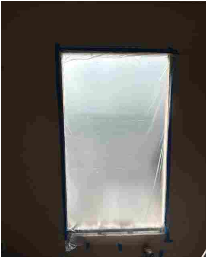
WINDOW INSTALLS BLDG 31
