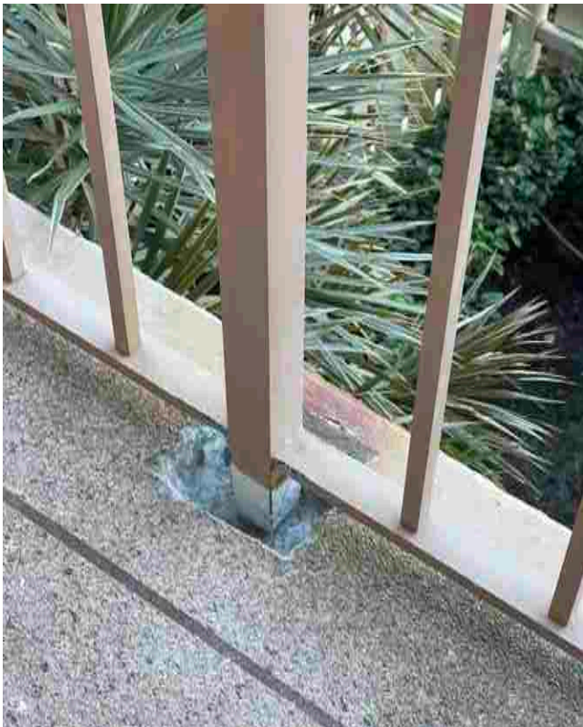
CHIPPING OF POST POCKETS BUILDING 31 SECOND FLOOR
