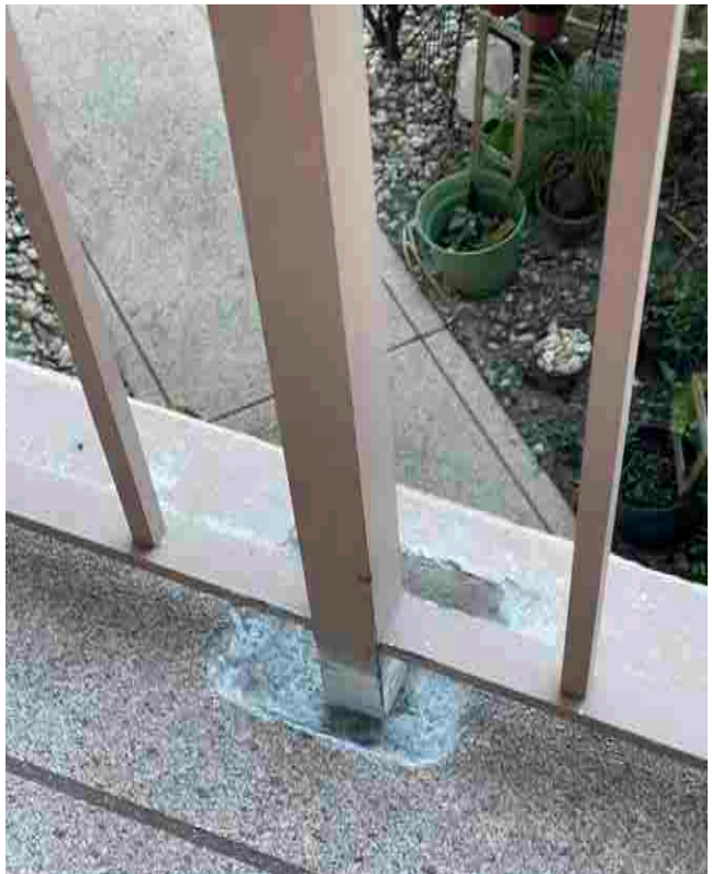
CHIPPING OF POST POCKETS BUILDING 31 SECOND FLOOR
