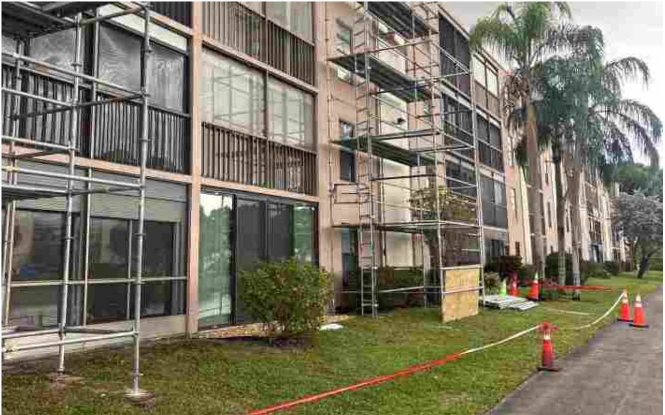
SCAFFOLDING INSTALLED ON BUILDING 31
