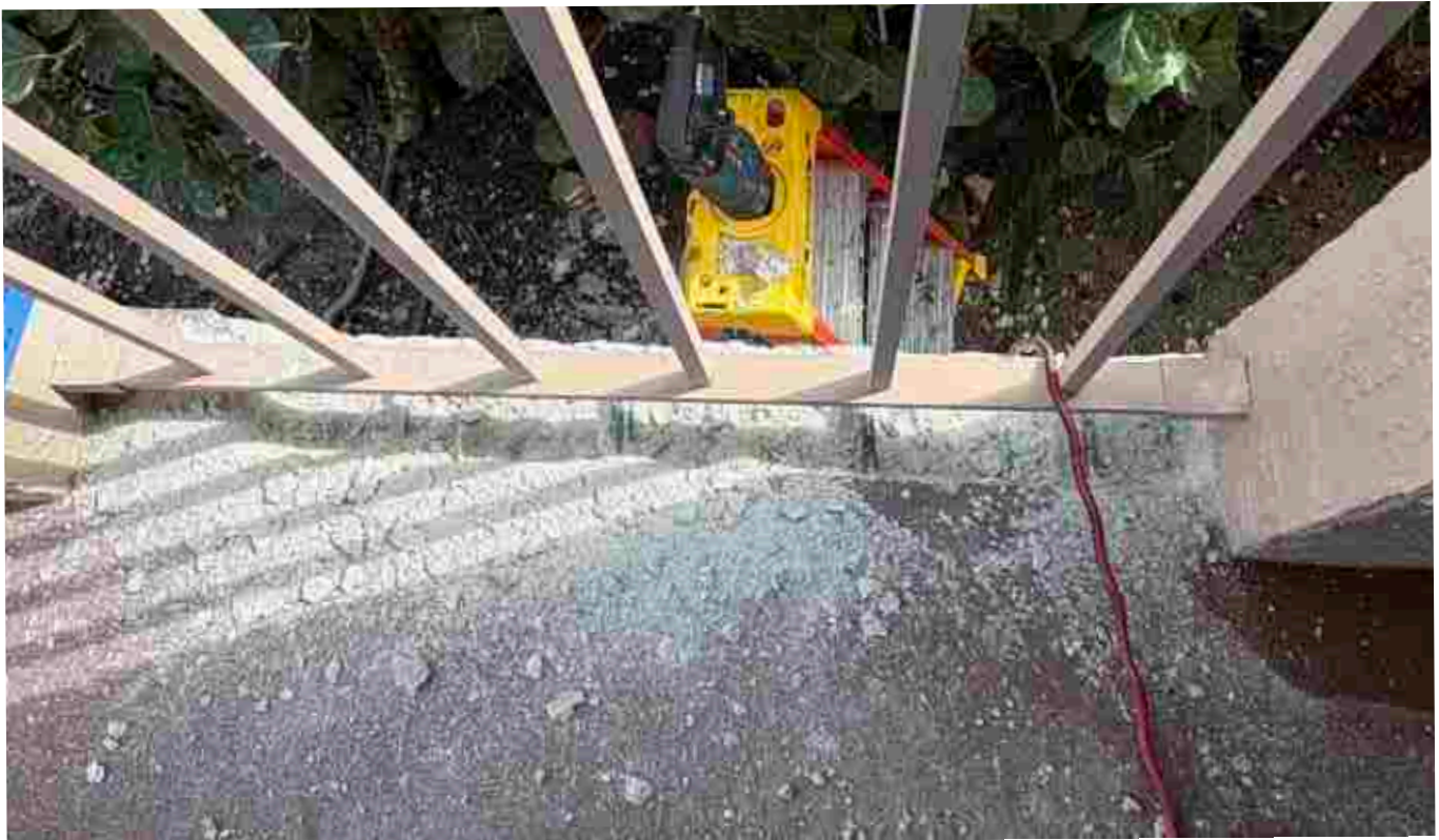
CHIPPING PARTIAL DEPTH EAST STAIRWELL
